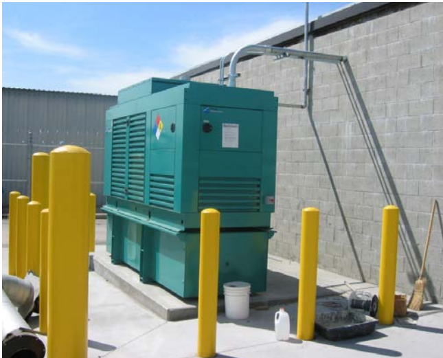
Figure 34. A typical emergency generator installation. Photo from Gladstein, Neandross & Associates, NREL 44689
