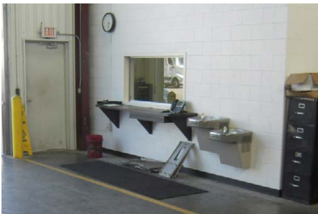
Figure 7. A pass-through window presents a potential path of migration. Photo courtesy of Gladstein, Neandross & Associates, NREL 44902
