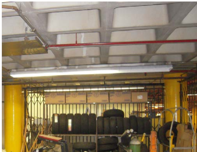
Figure 13. Ceiling configuration with “pockets.” Photo courtesy of Gladstein, Neandross & Associates, NREL 44704
