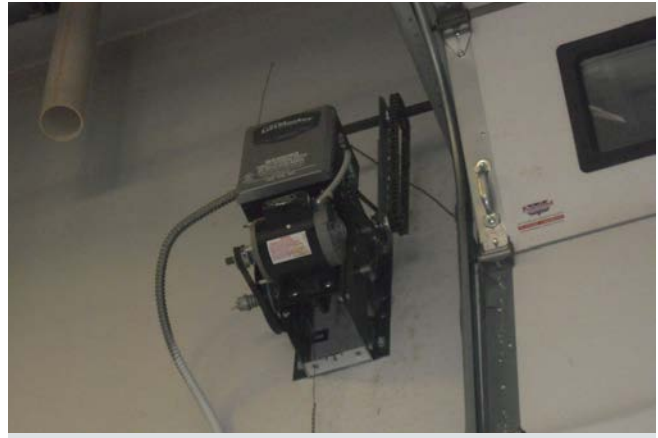
Figure 26. A typical electric door motor. Photo from Gladstein, Neandross & Associates, NREL 44680
