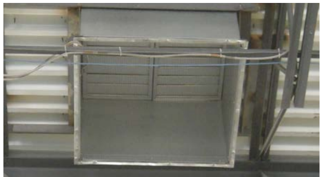
Figure 9. Direct fan intake with louvers. Photo courtesy of Gladstein, Neandross & Associates, NREL 44700
